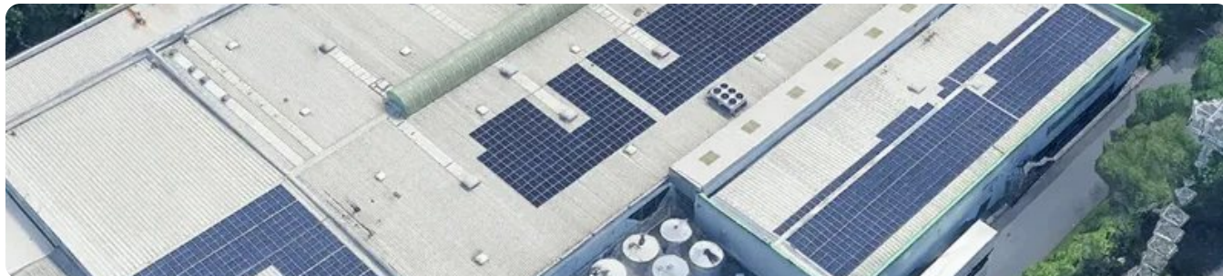
On-site solar generation at Olympic's Merseyside production facility.
